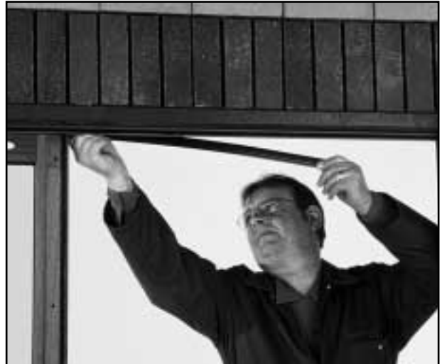
19 Remove the short locating bar and slide into the fixed door top rail and, tap home.
