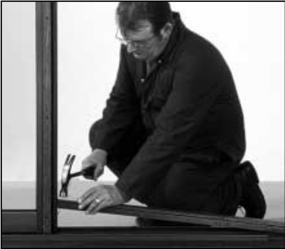
37 Fit threshold into place and screw down.
