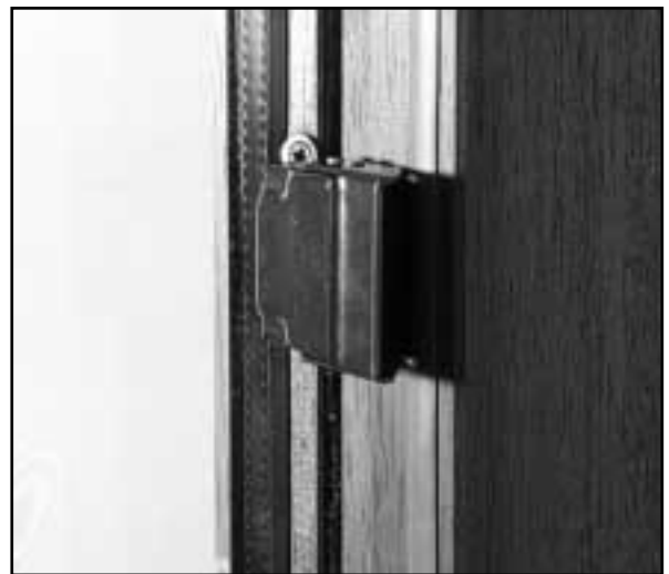
42 Catch correctly fitted.
