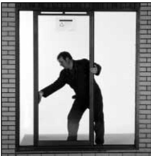
18 Slide the fixed door until it locates onto the side locating bar.
