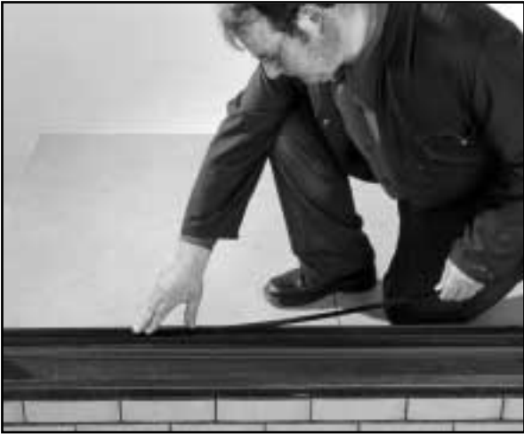
16 Lay the short locating bar on the inside of the sill on top of foam tape as a temporary packer to avoid damaging the foam seal when placing fixed door in position.
